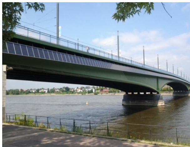
Solar panels along the river bridge in Bonn
